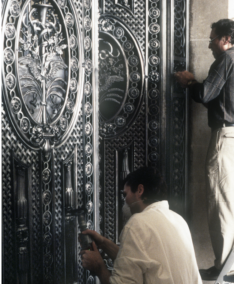
Figure 11.16b Cleaning the Grille in the Louvre Museum, cast and forged iron, France, ca. 1646-1650 (photograph by Carol Ventura, 2009).
